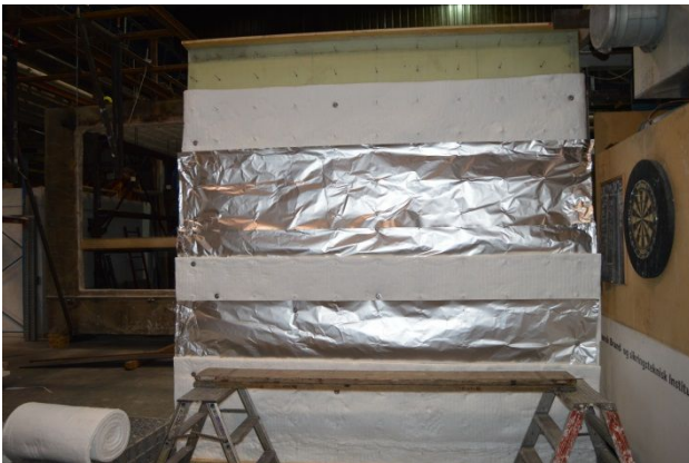
The FRP bulkhead as it is getting insulated.
